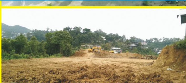
YRC hmun laih mek chu ruahsur avanga hun eng emaw chen chawlsan a nih hnuin August 5, 2015 atang khan laih chhunzawm a ni leh ta. Excavator lian 1 leh JCB 2 in lain Tripper 5 leh LPK 11 ten an an paih thin.
