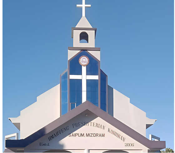
Saipum Hmarveng Church constructed in partnership with Dawrpui Church
